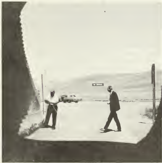
Looking East from EAST ENTRANCE
